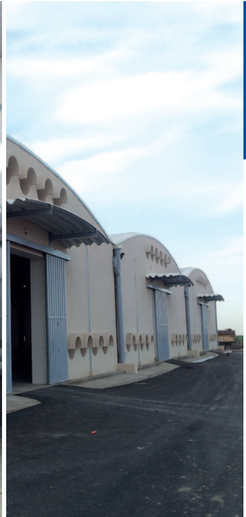
Turnkey Processing Lines
